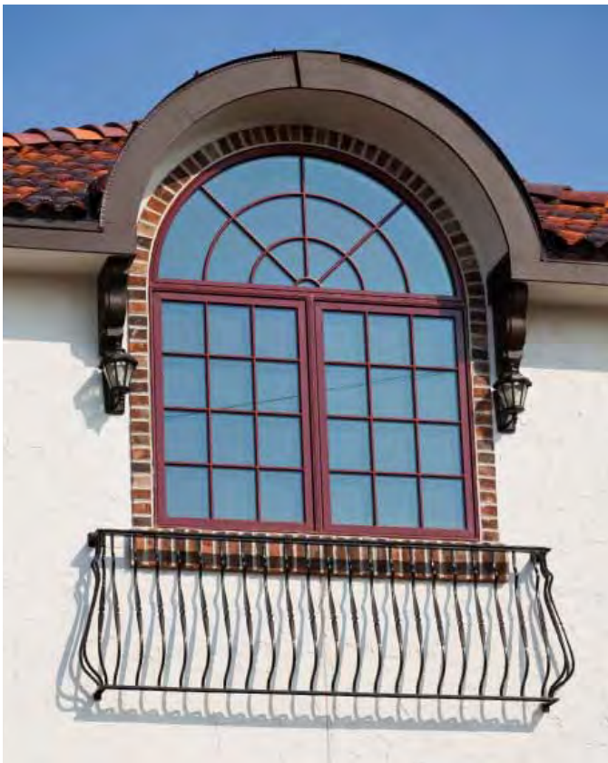
Manchester railing creating a French balcony, Longport, NJ
