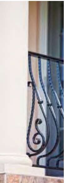
Close-up of scroll for code compliance
