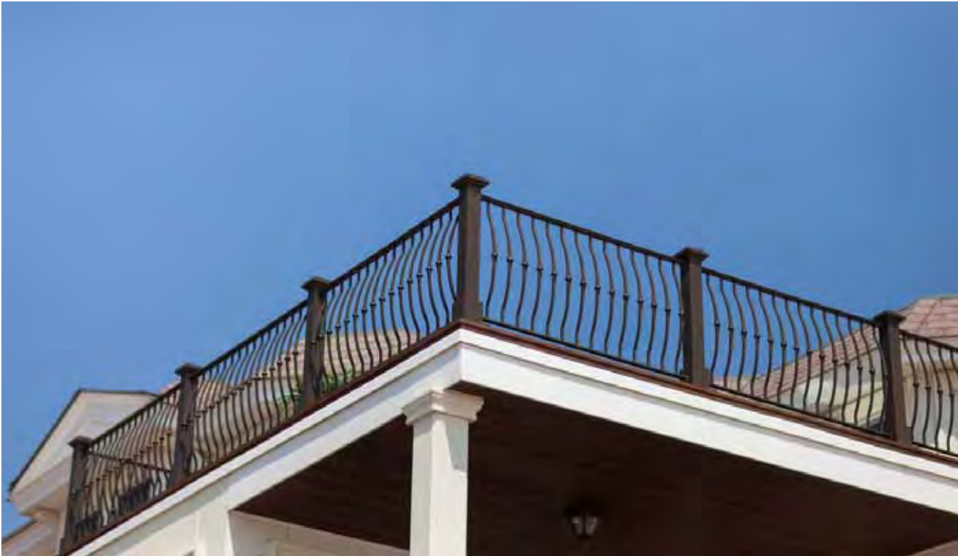
Terrace railings and posts have a cohesive effect for this shore home
