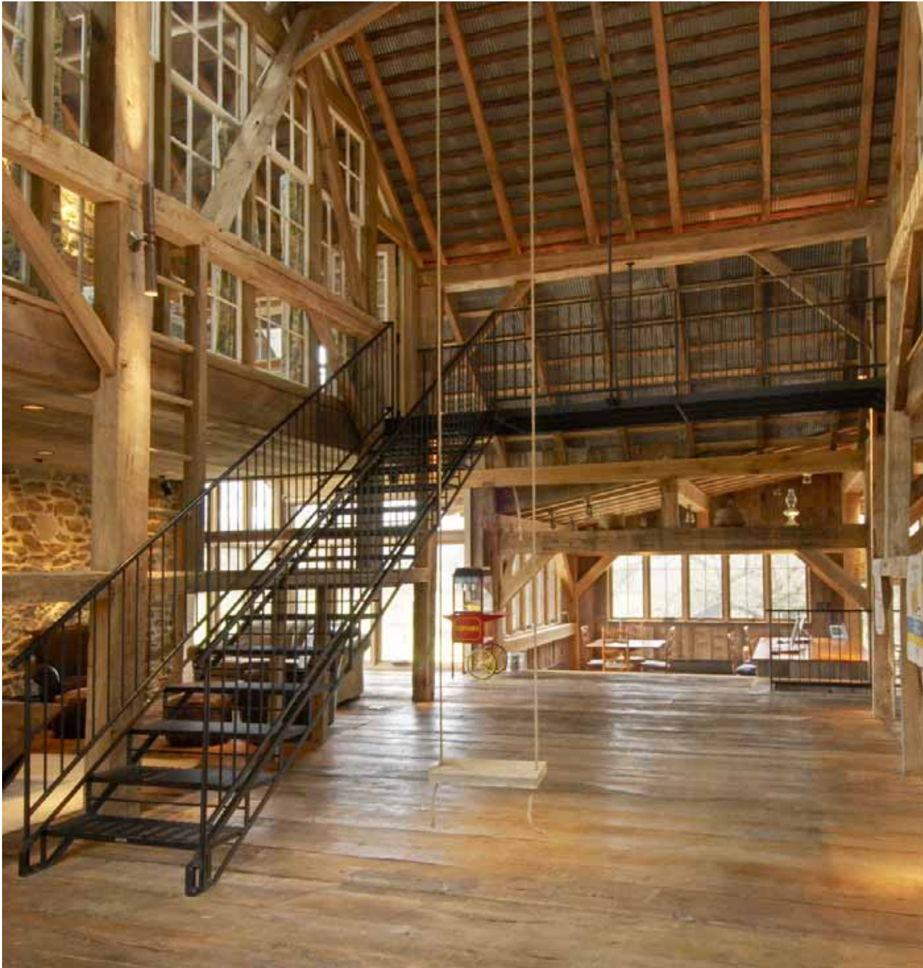
Custom stairs and hallway in 1840s barn, refurbished into a house
