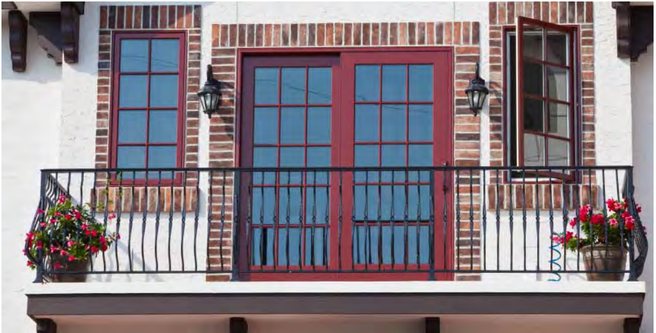
Manchester railing on Romeo balcony in Longport, NJ
