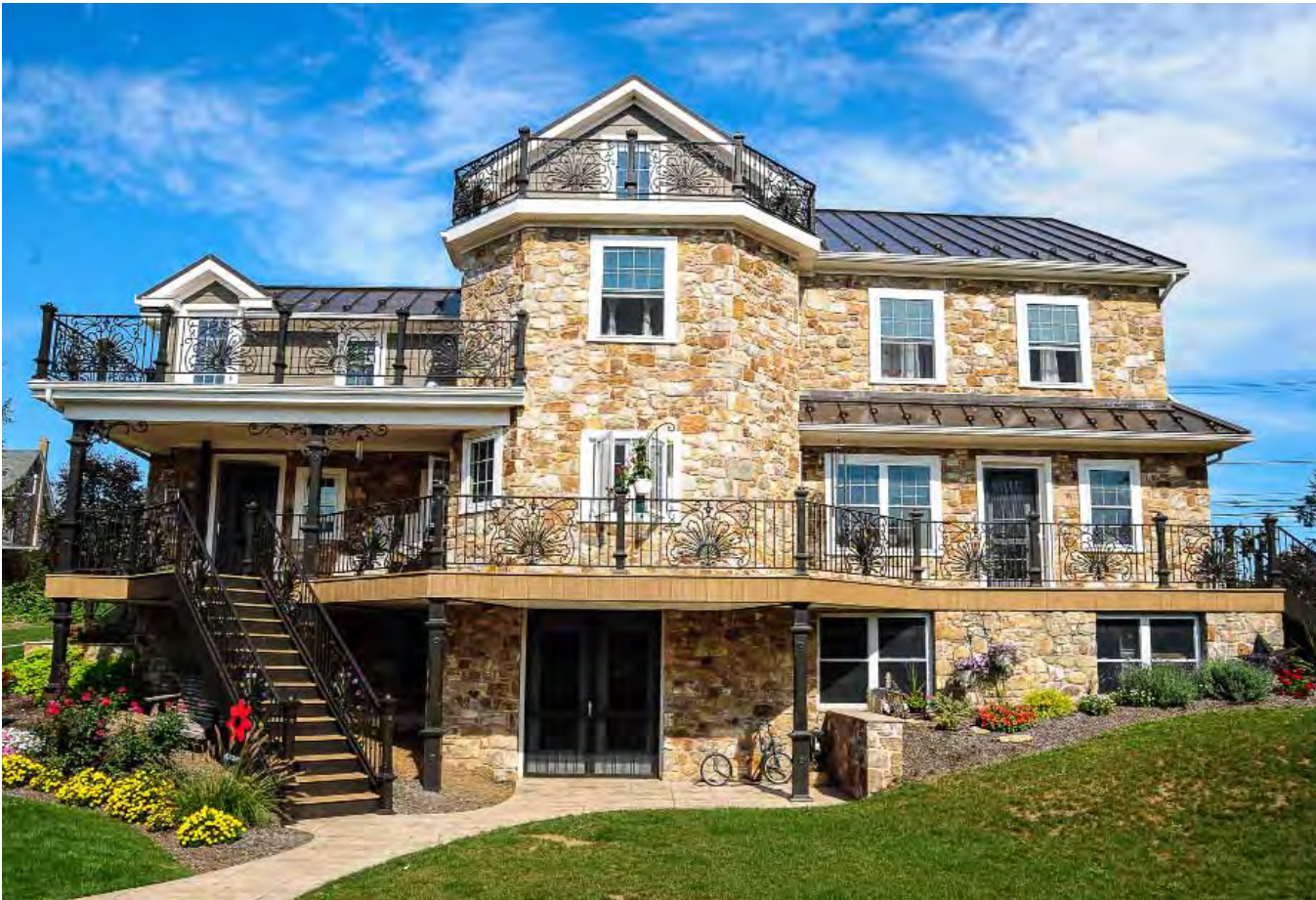
3 Levels of forged aluminum railing indistinguishable from wrought iron
