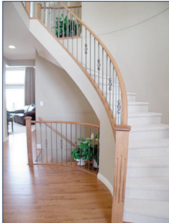
Builders Line Western; Plywood Treads and Closed Plywood Risers.
