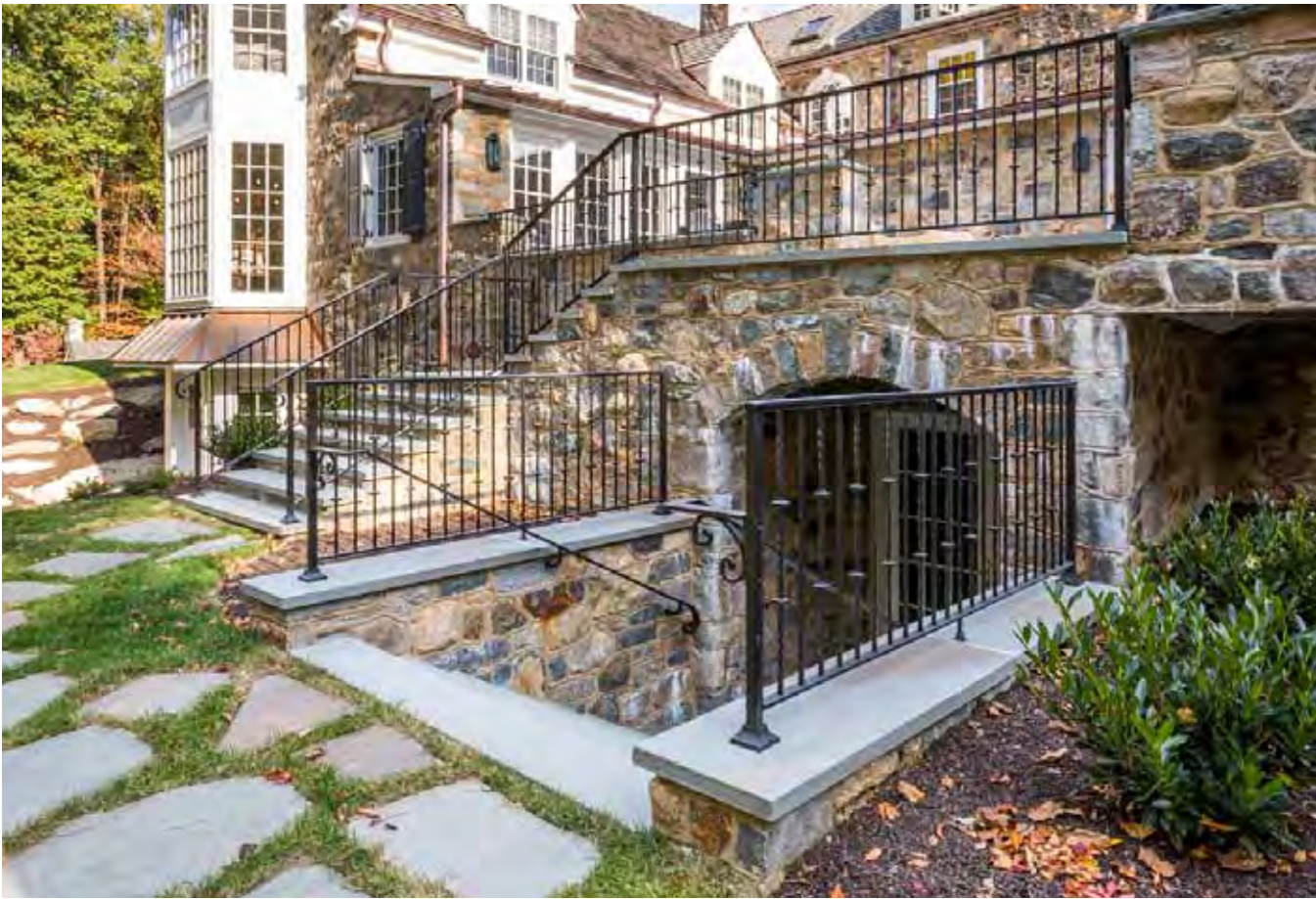
Wrought iron railing specially created with todays materials for an authentic look
