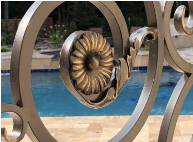
Detail of forged rosette and leaf for stair railing
