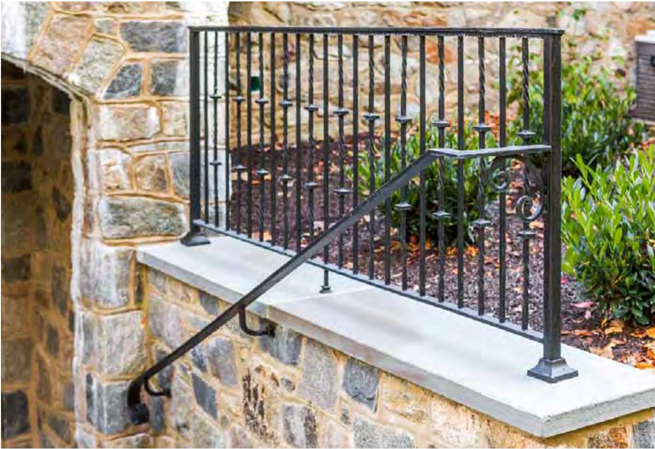
Metal handrail for stairs and safety railing
