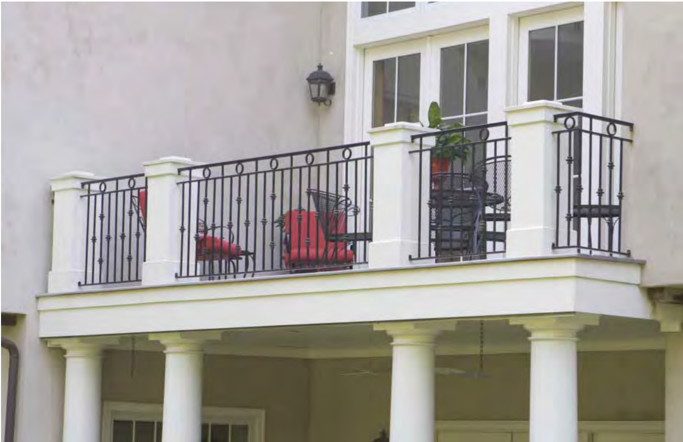
Mainline terrace railing
