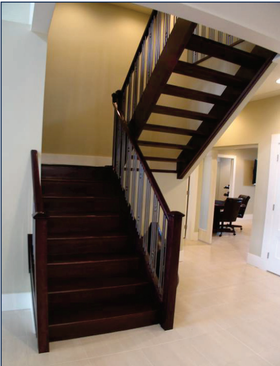
Both: Full Westerns; Veneered Stringers Upper: Solid Treads, Open Risers Lower: Solid Treads, Closed Risers.
