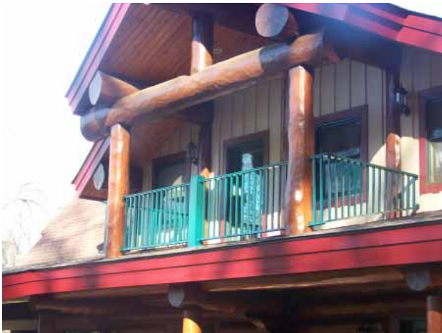
Custom railing to match the decor of a log home in Washington, NJ
