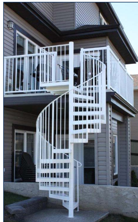
Exterior Spiral Stairs
