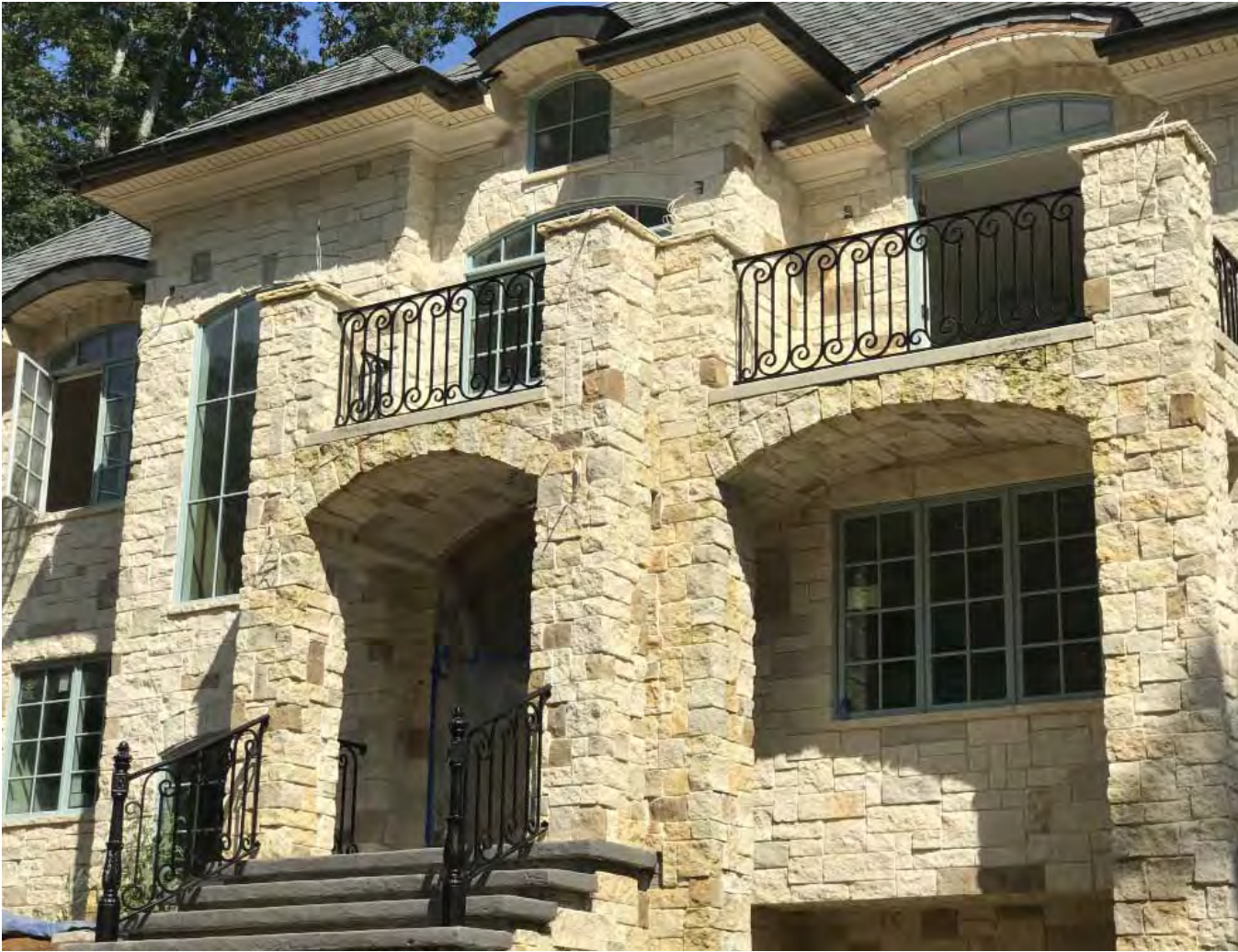
House railing in contemporary materials
