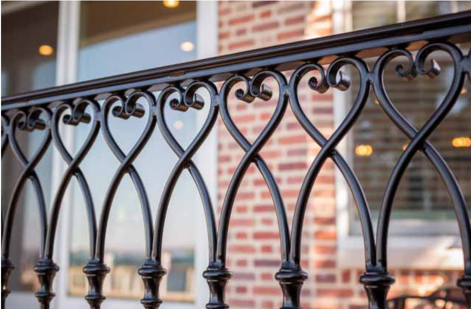
Close up of wrought iron railing design
