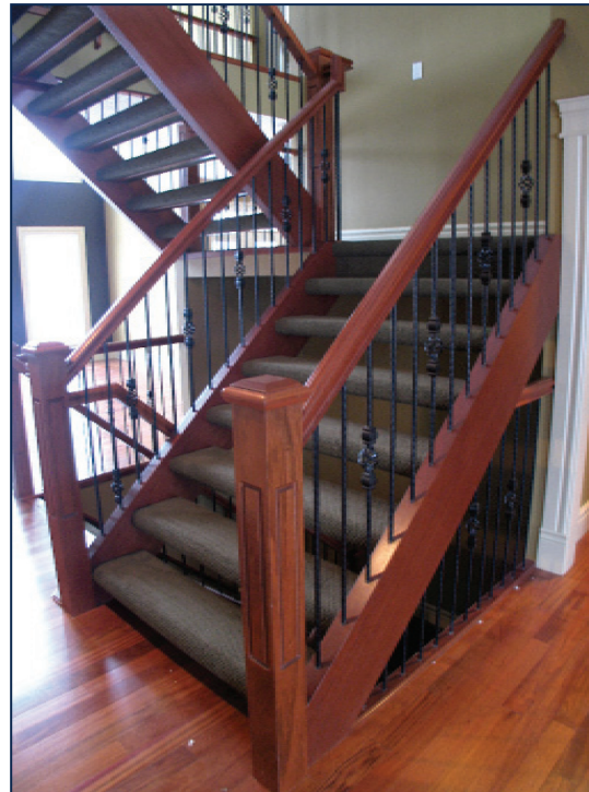
Full Westerns; Veneered Stringers; Plywood Treads and Open Risers Complete with Carpet Tees.
