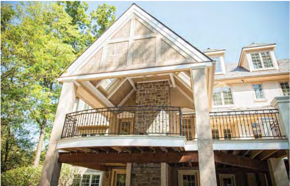
Mainline railing on a radiused terrace
