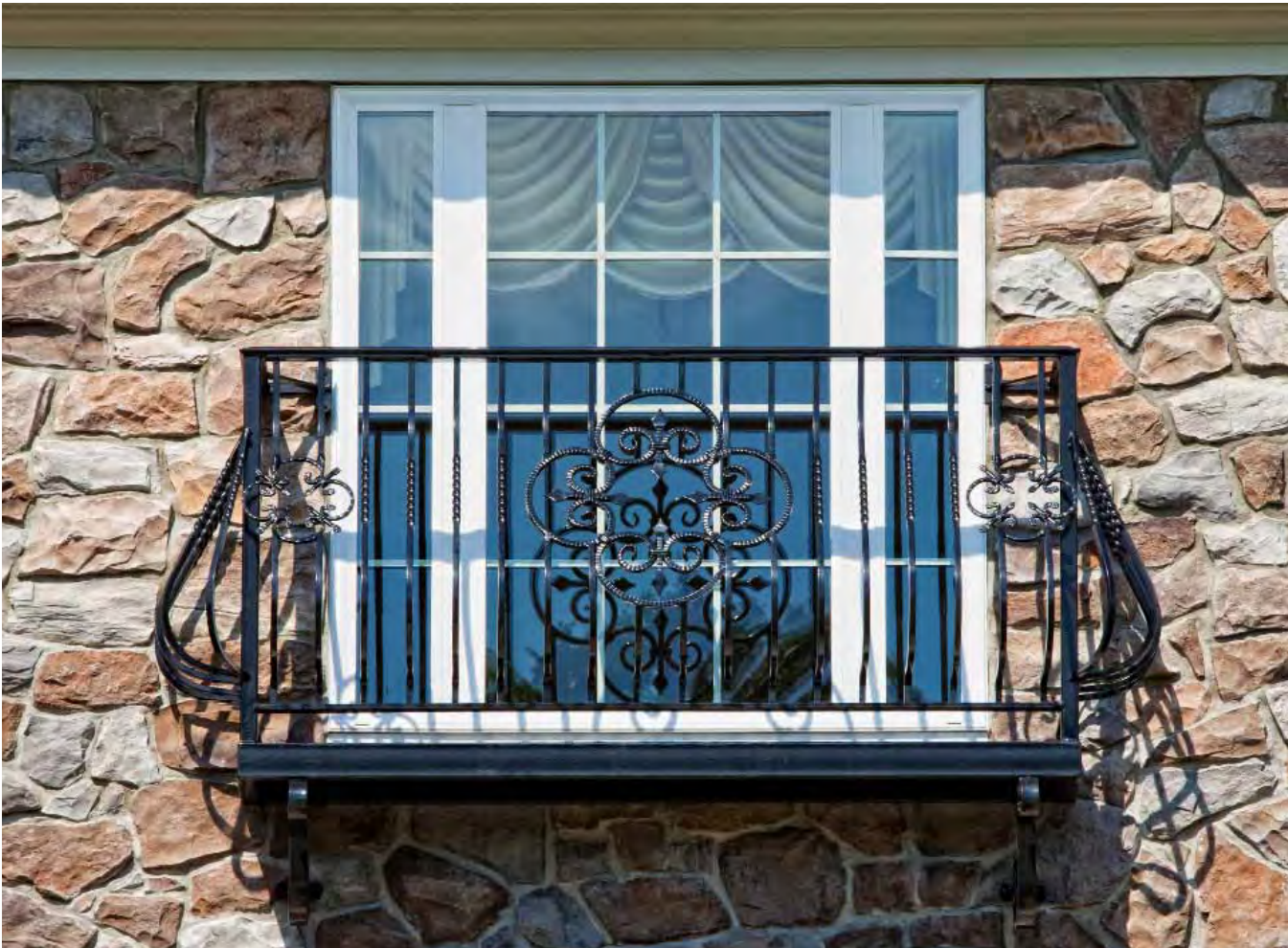
Tewksbury railing with rosette on Juliet balcony in Downingtown, PA
