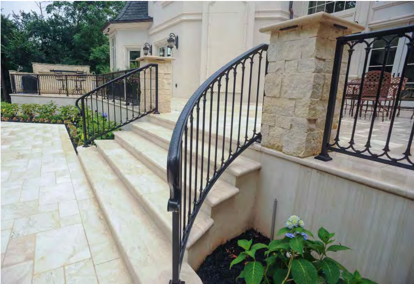
Custom castings were created for the angle of these stair railings
