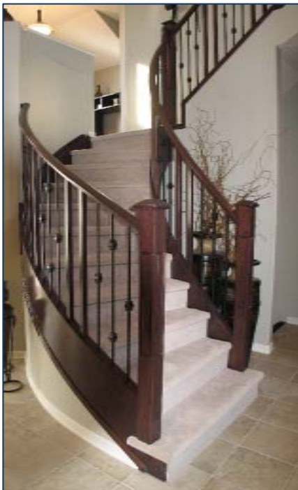
Full Western; Veneered Stringer; Plywood Treads with Carpet and Closed Plywood Risers.
