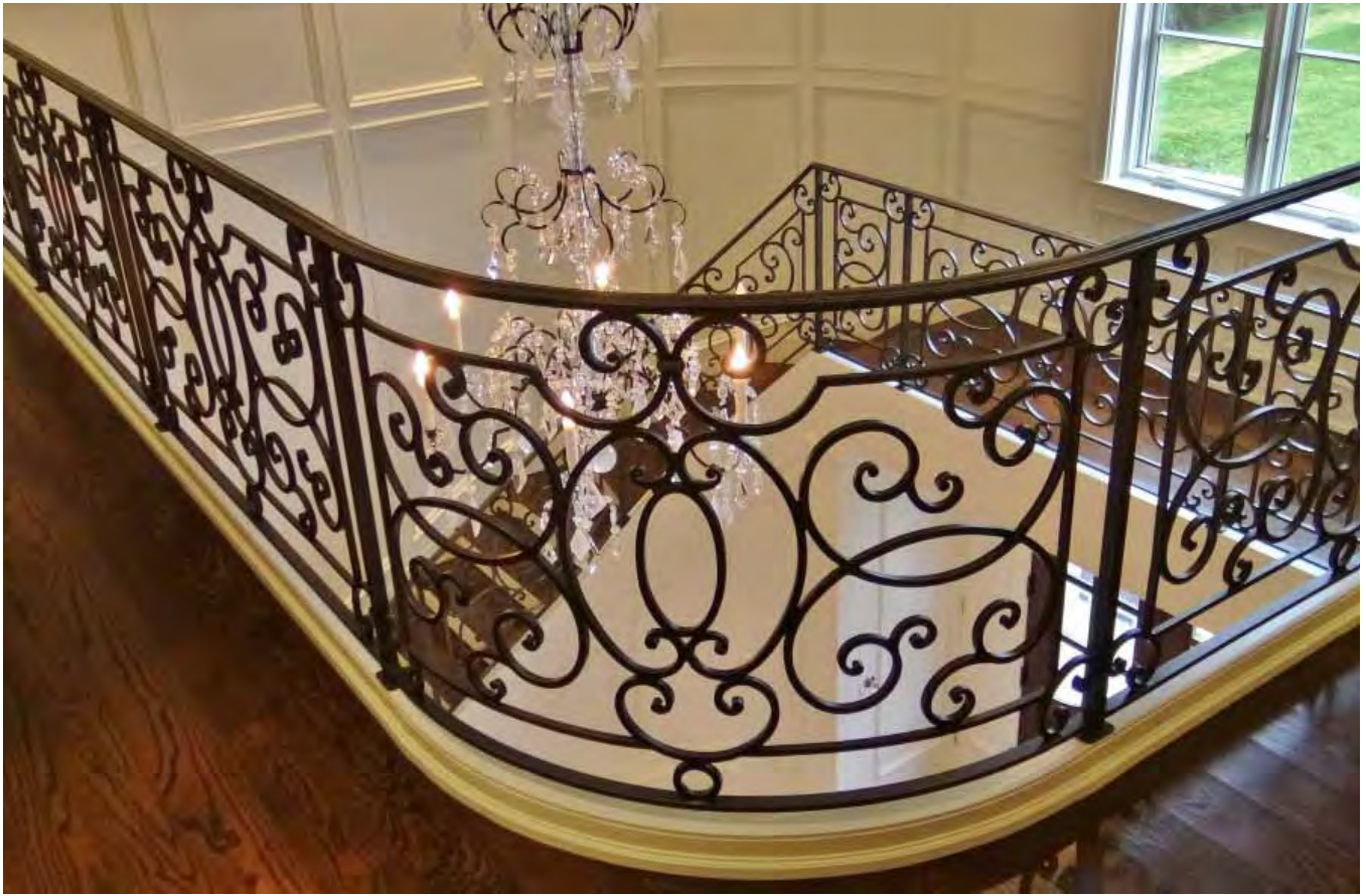
Overview of interior iron railing
