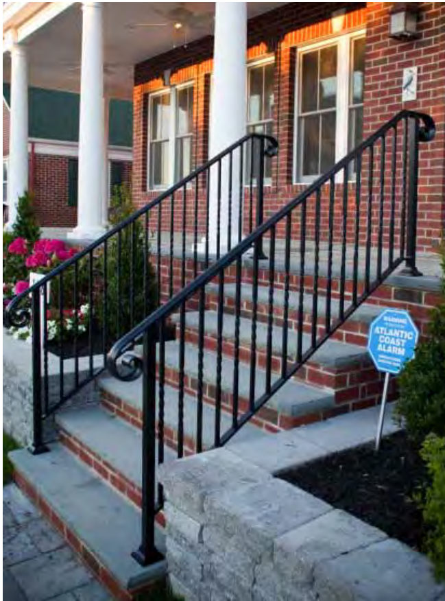
Tewksbury stair railings in Margate, NJ
