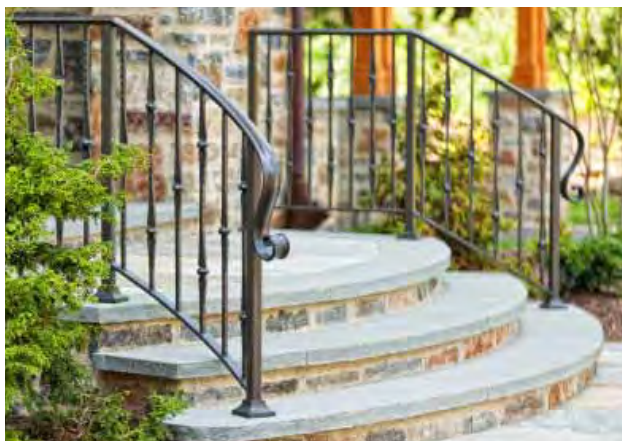
Custom entry railing in Bryn Mawr, PA
