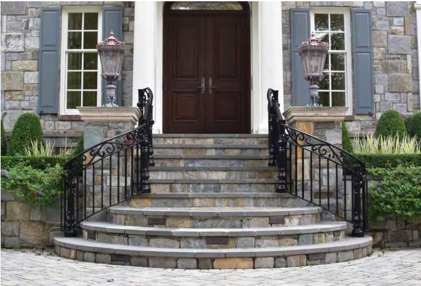
Both sides of entry railing provide symmetry for front stairs
