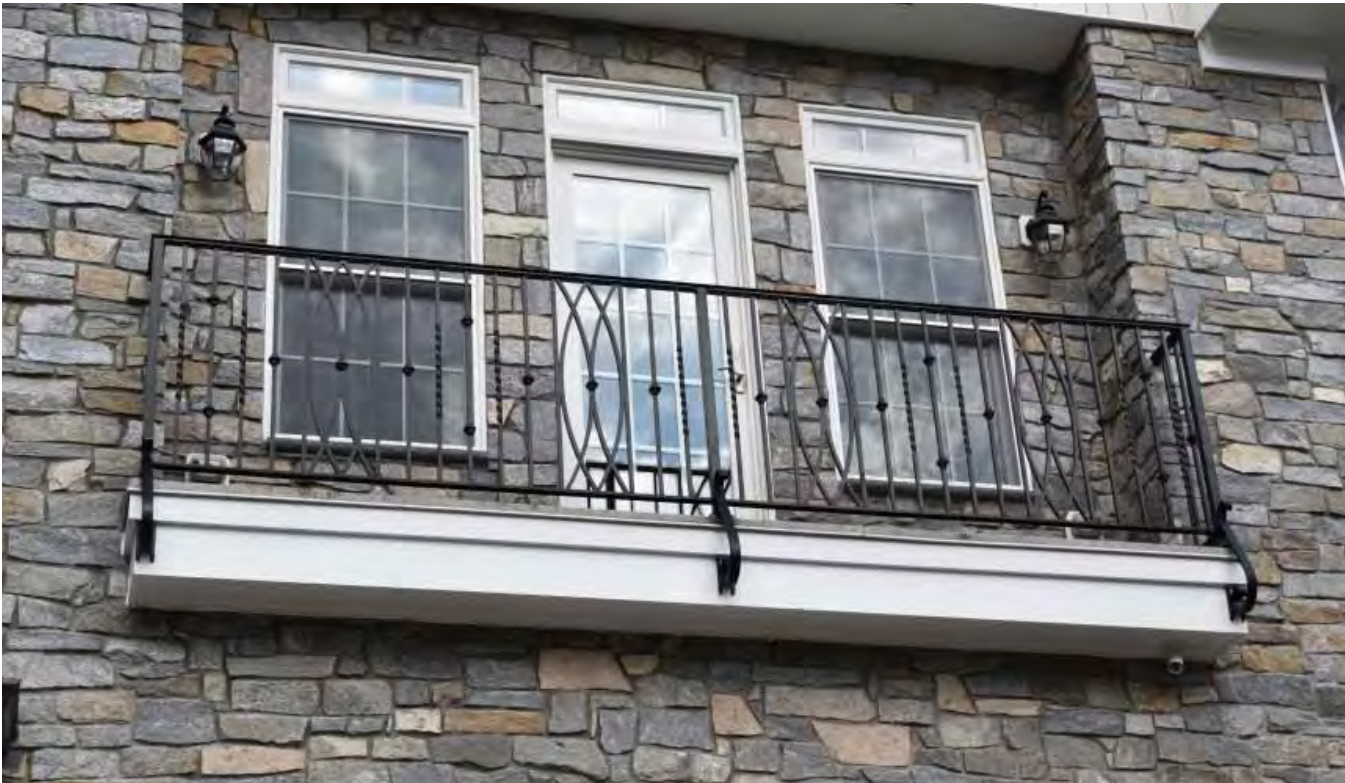
Balcony railing in aircraft grade aluminum
