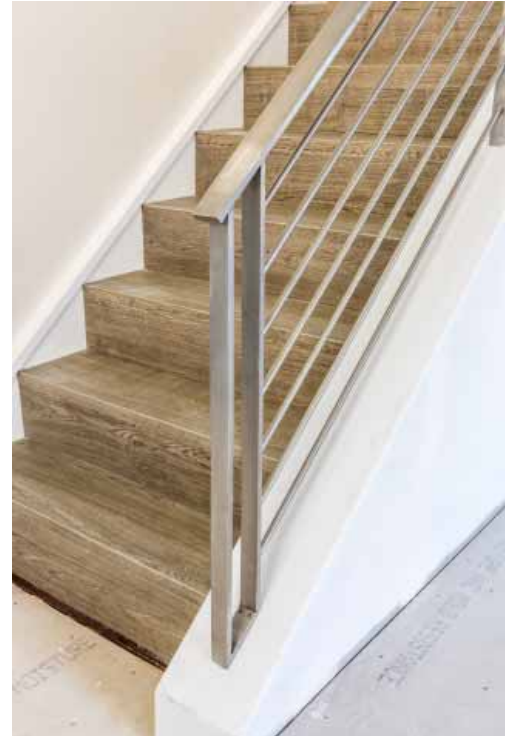
The contrast of flat bar and round bar in stainless for a contemporary look
