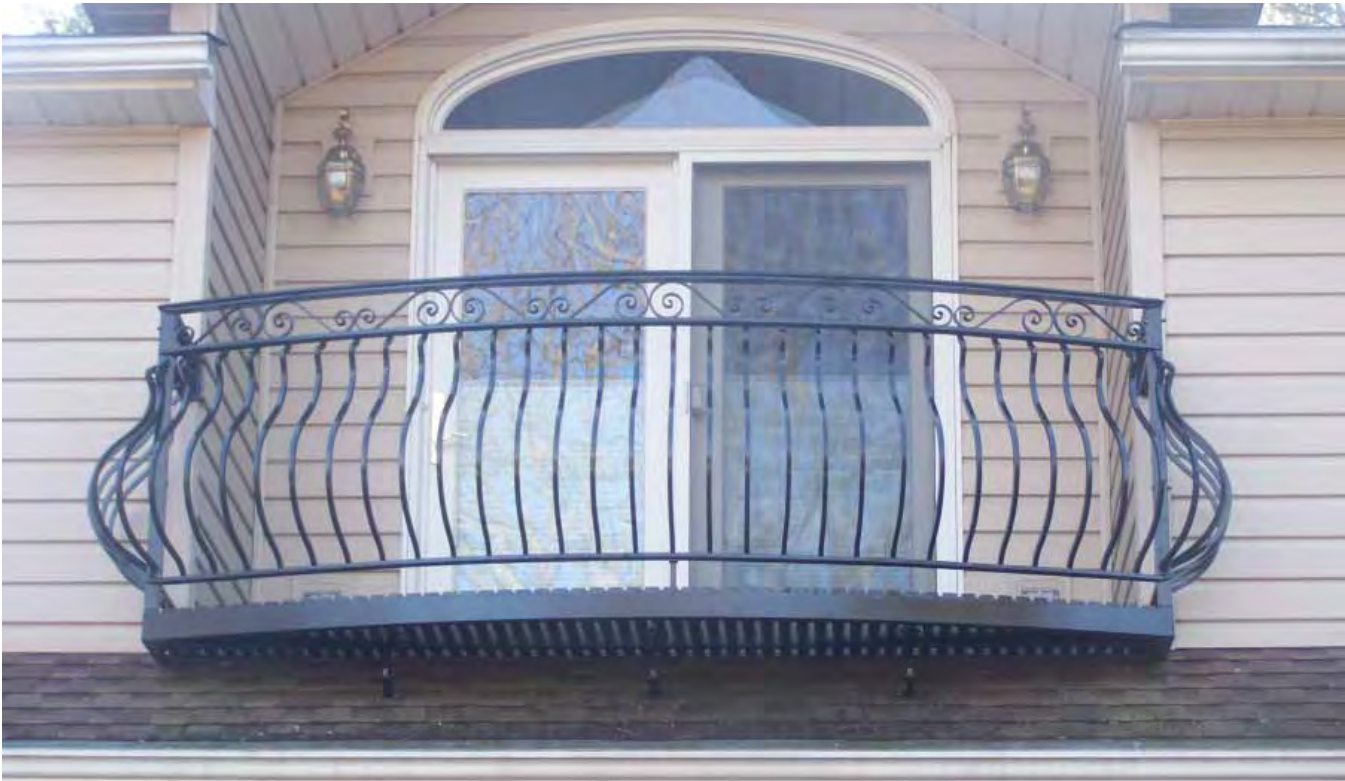
Solid aluminum railing on Juliet balcony in Chester County, PA
