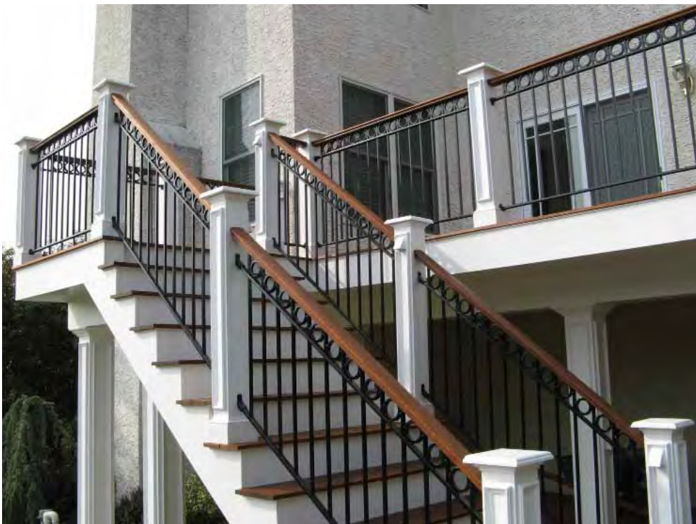
Custom iron railing with IPE handrail in West Chester, PA
