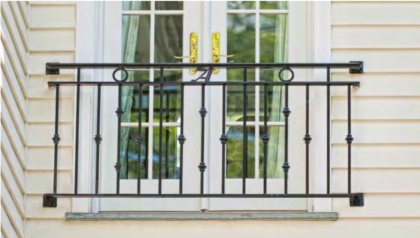
Mainline style French balcony in Villanova, PA
