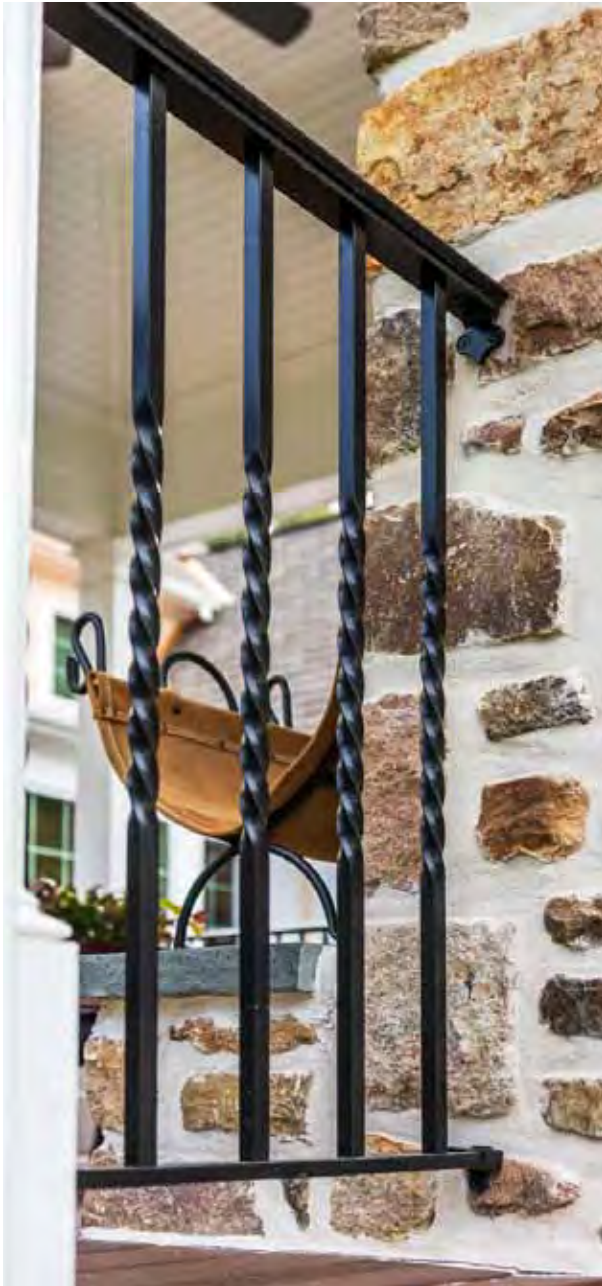
Terrace railing attachment to masonry
