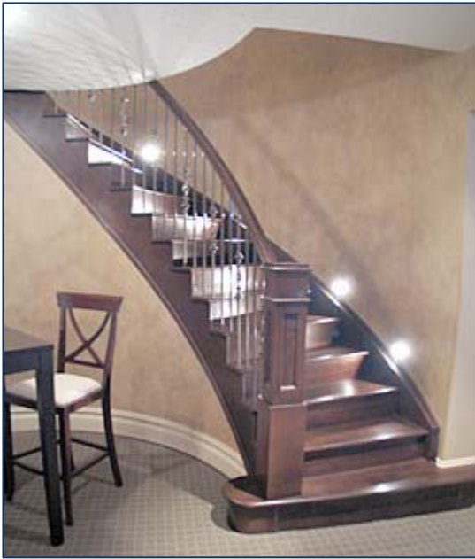
Full Eastern (with Western Wall Stringer) Veneered Stringer; Solid Treads and Closed Risers.
