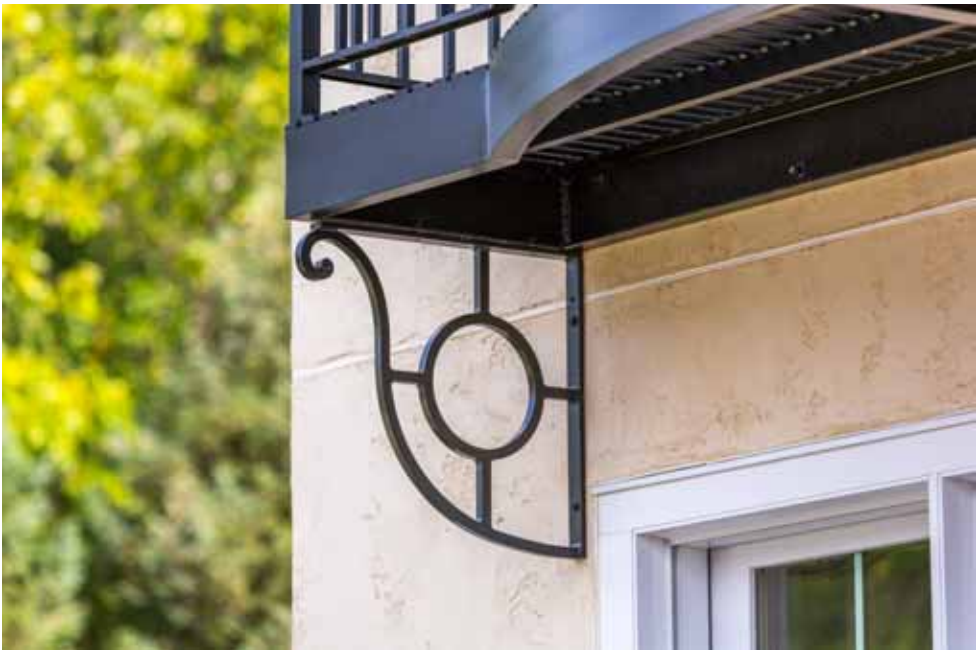
Brace detail for balcony and railing
