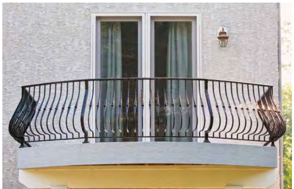
Hampshire Belly railing on bedroom terrace
