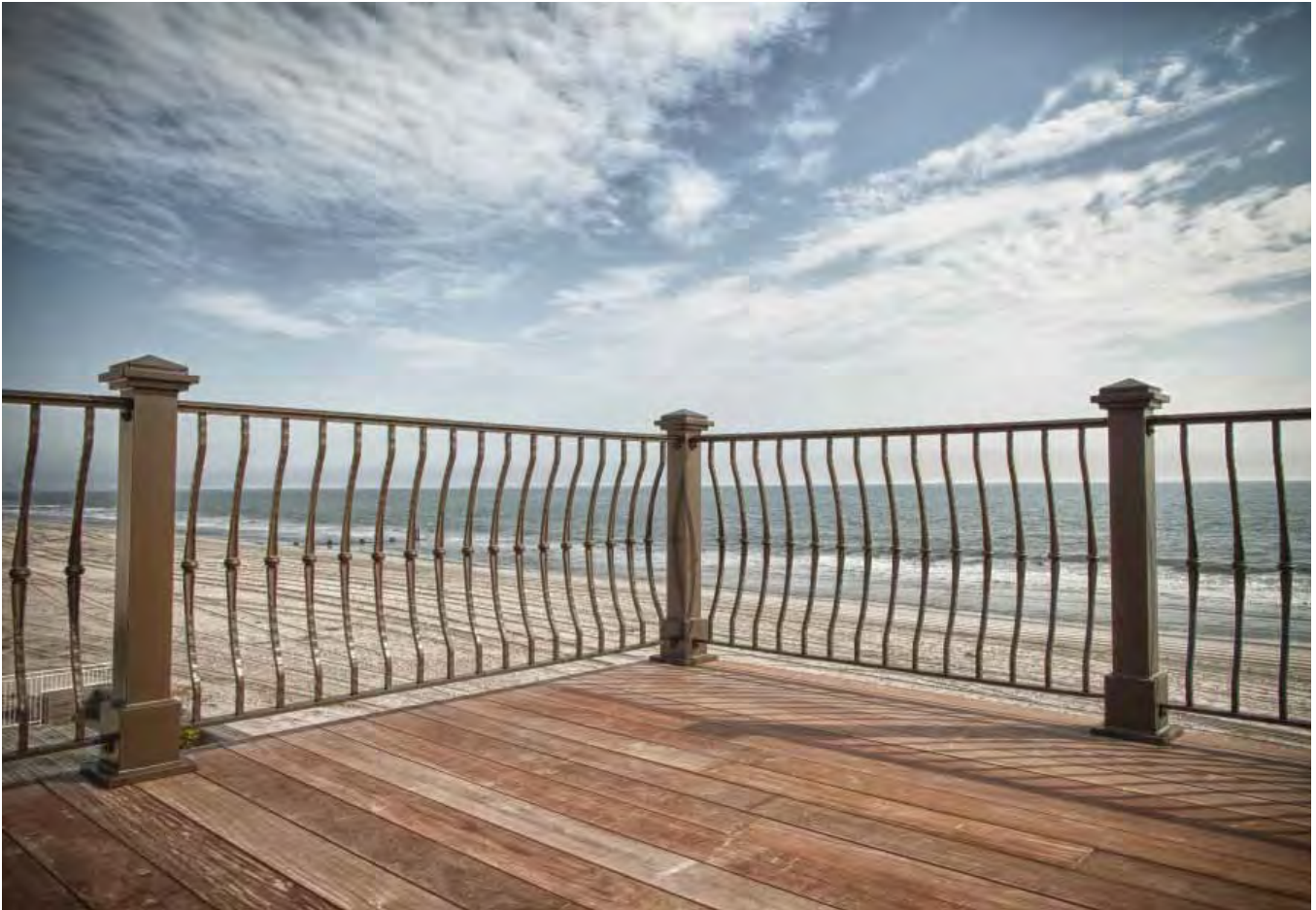
Custom aluminum railing withstood Hurricane Sandy
