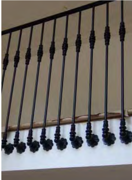
Level rail with custom forged balusters
