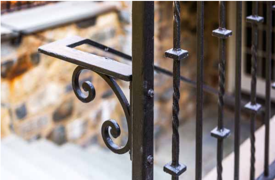
Close up of Iron railing that has an antique iron paint process to look like it was built decades ago
