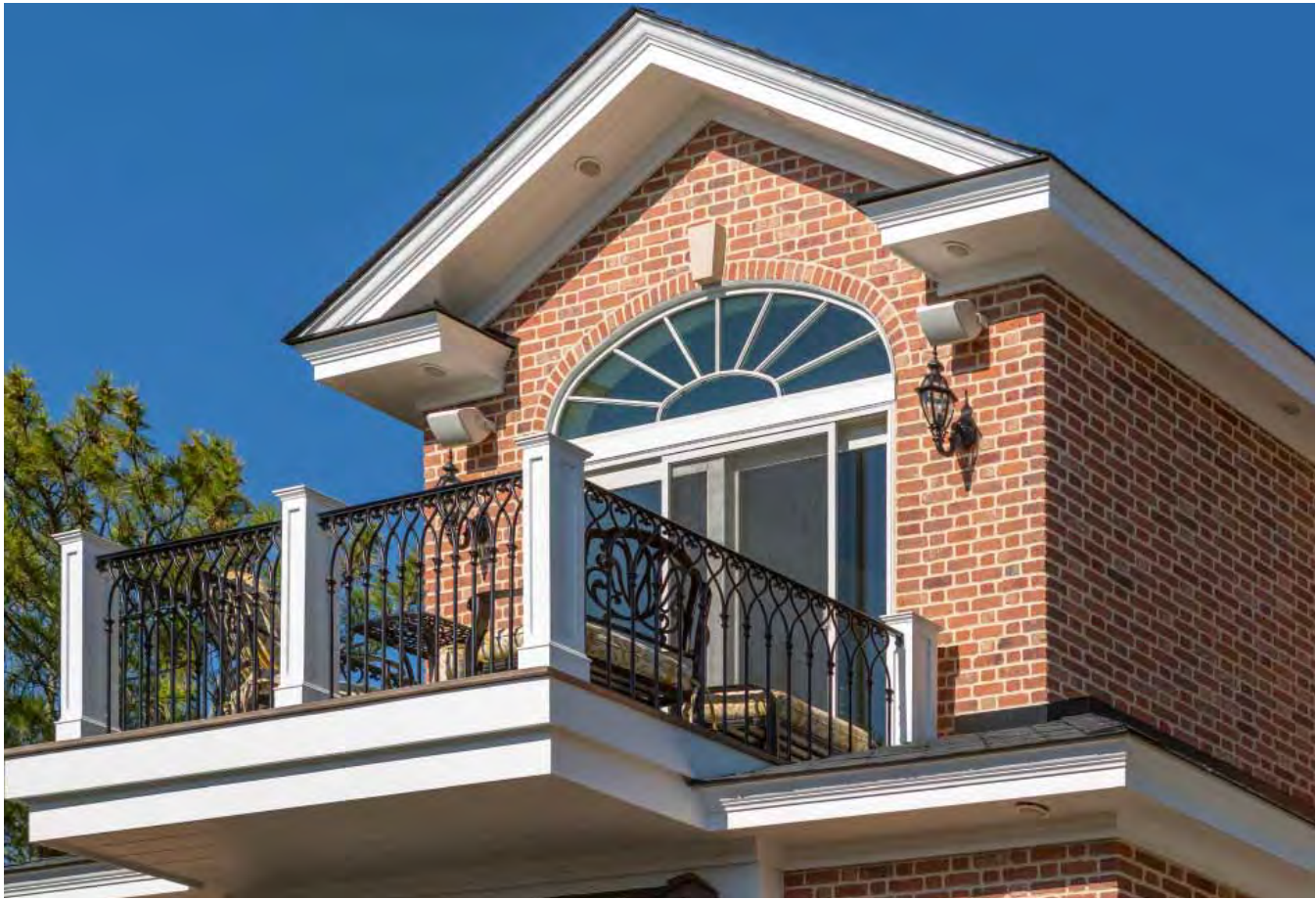
Exterior balcony railing forged from aircraft grade aluminum, indistinguishable from wrought iron
