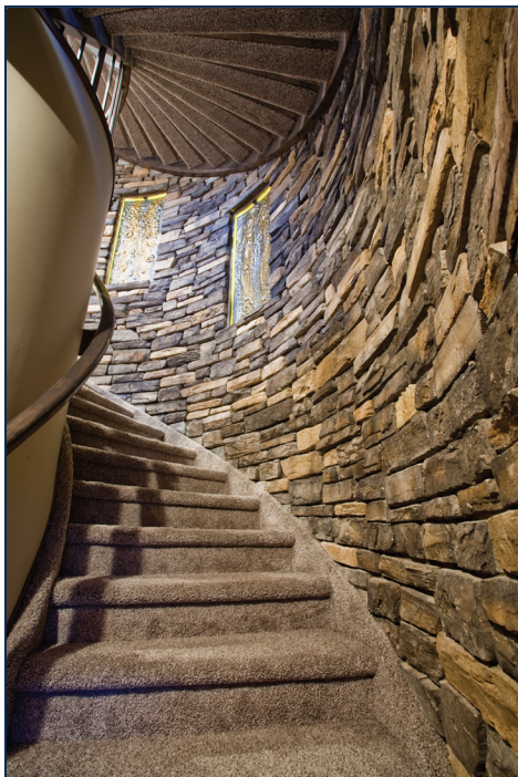
Builders Line Western; Plywood Treads and Closed Plywood Risers; Between Walls.
