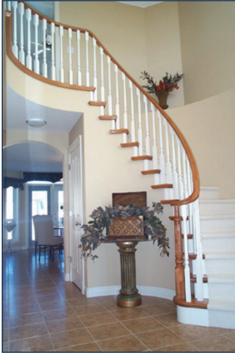
Builders Line Eastern; Plywood Treads and Closed Plywood Risers; Tread Caps installed on Inside Radius.
