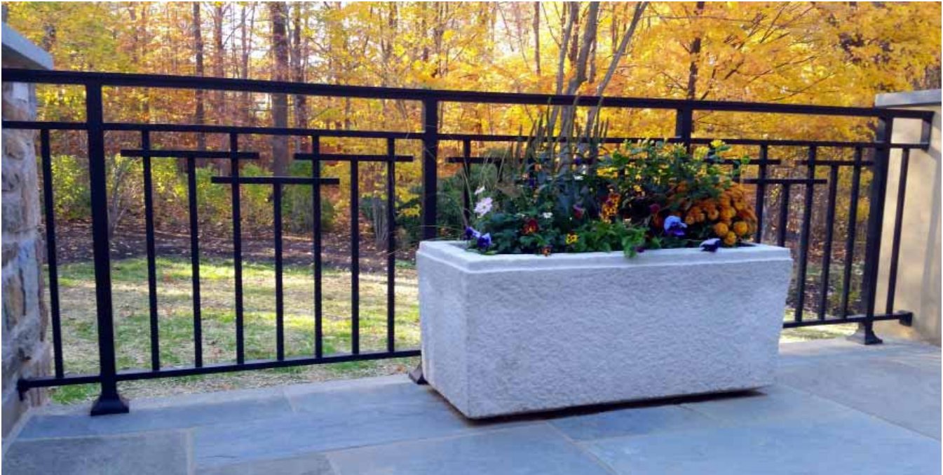
Arts and crafts style railing in solid aluminum displays a taste of progressive design.
