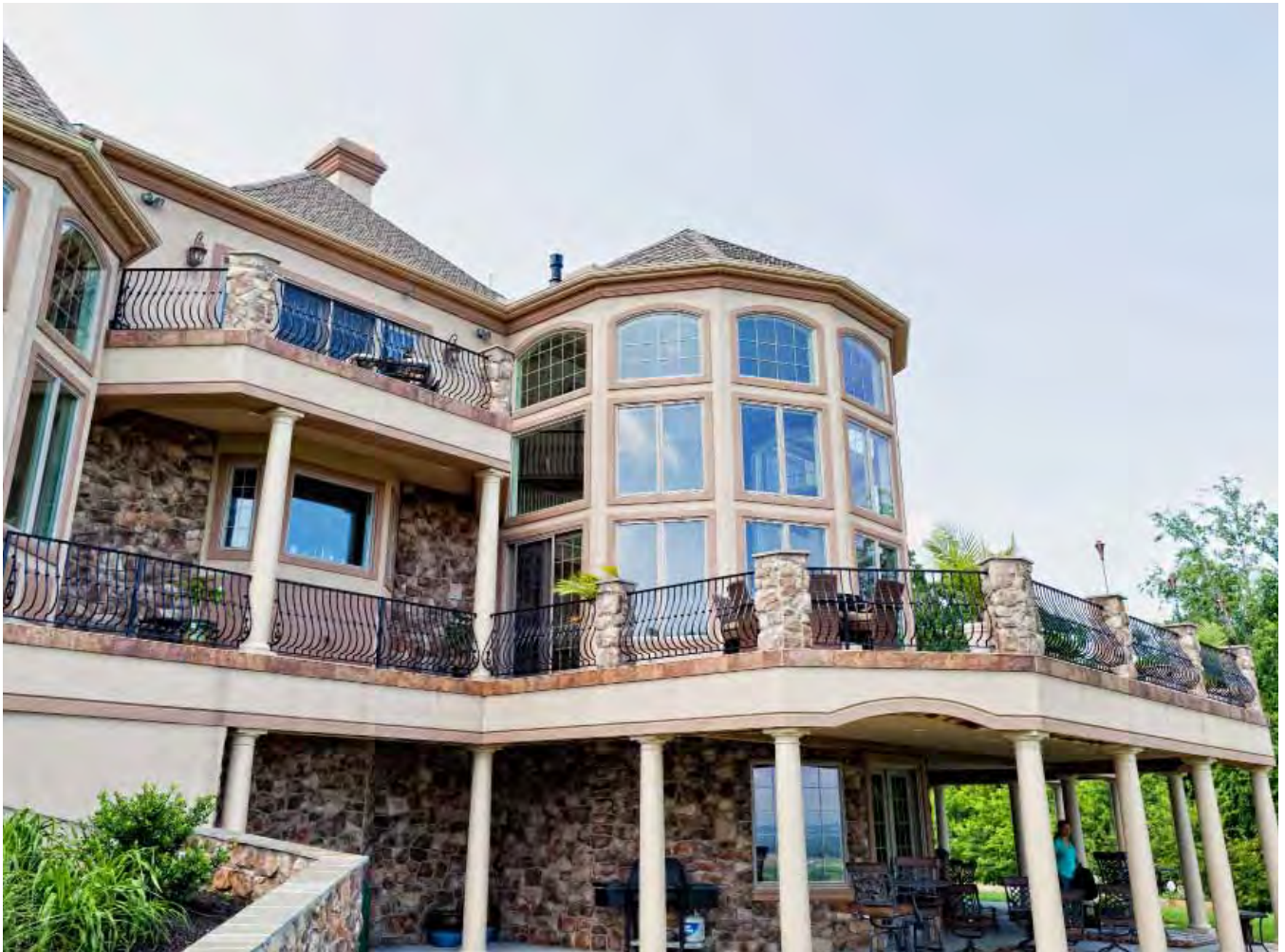
Hampshire Belly railing in Lebanon, PA
