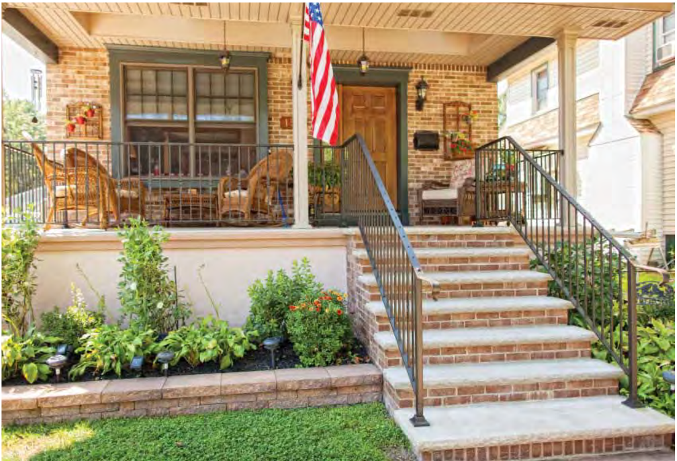
Roanoke railing is a solid match for this brick home
