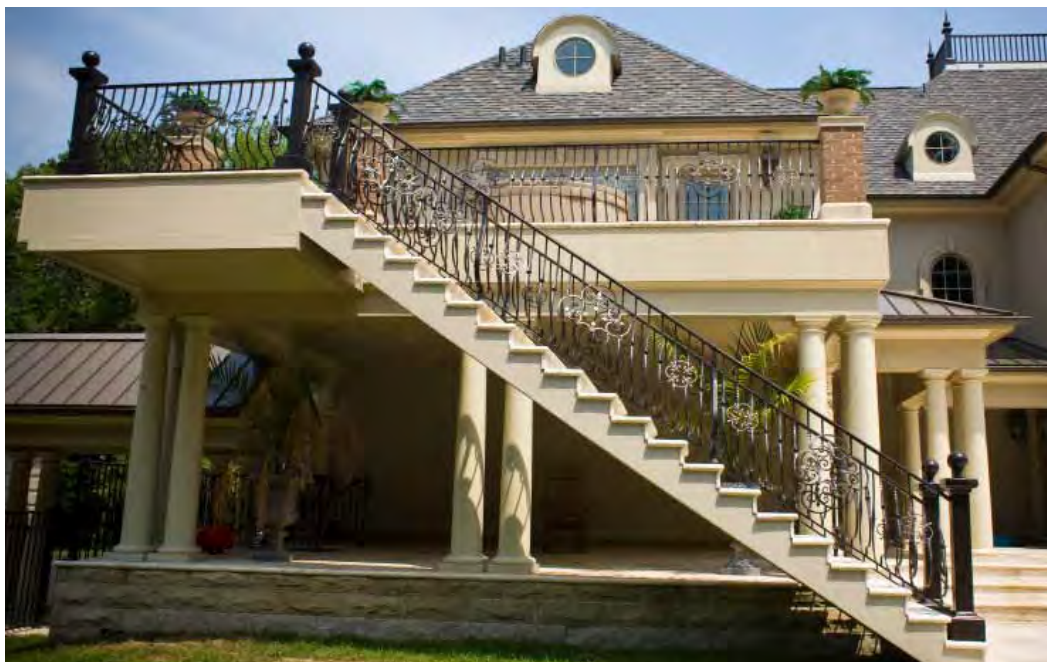
Terrace step railings in Moorestown, NJ
