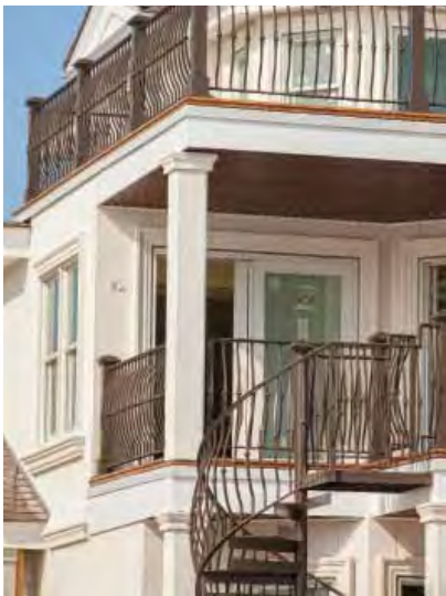
Custom spiral stair matches terrace railing
